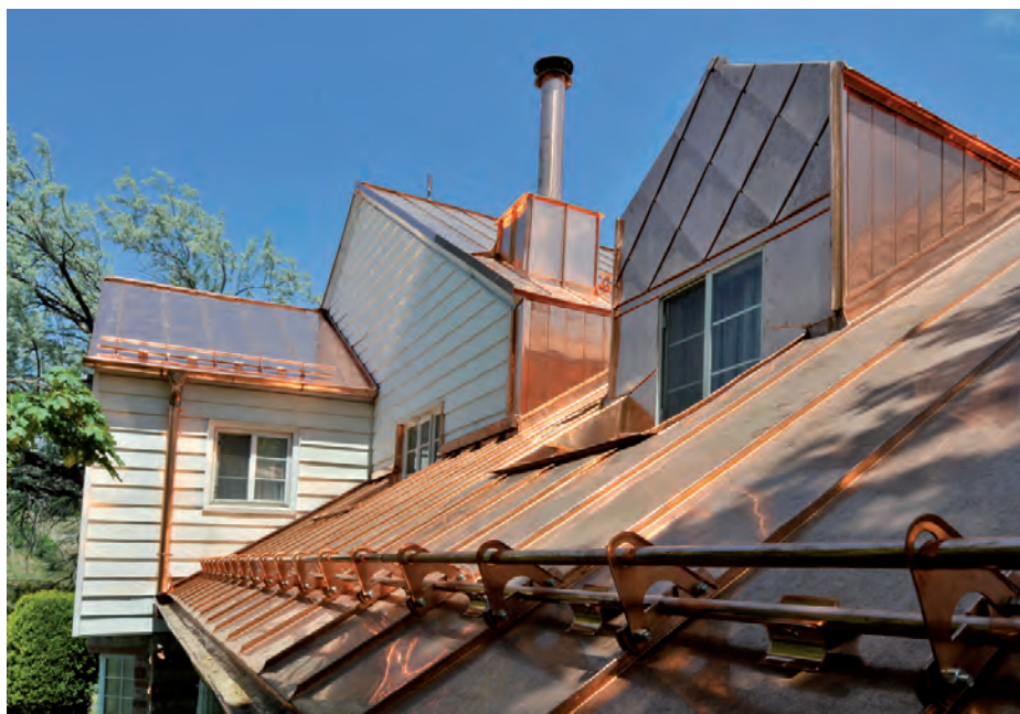
Pict. 2: The gutter board tubes shown here are made of copper. They are fastened by copper clamping lugs on the standing seam roof.
